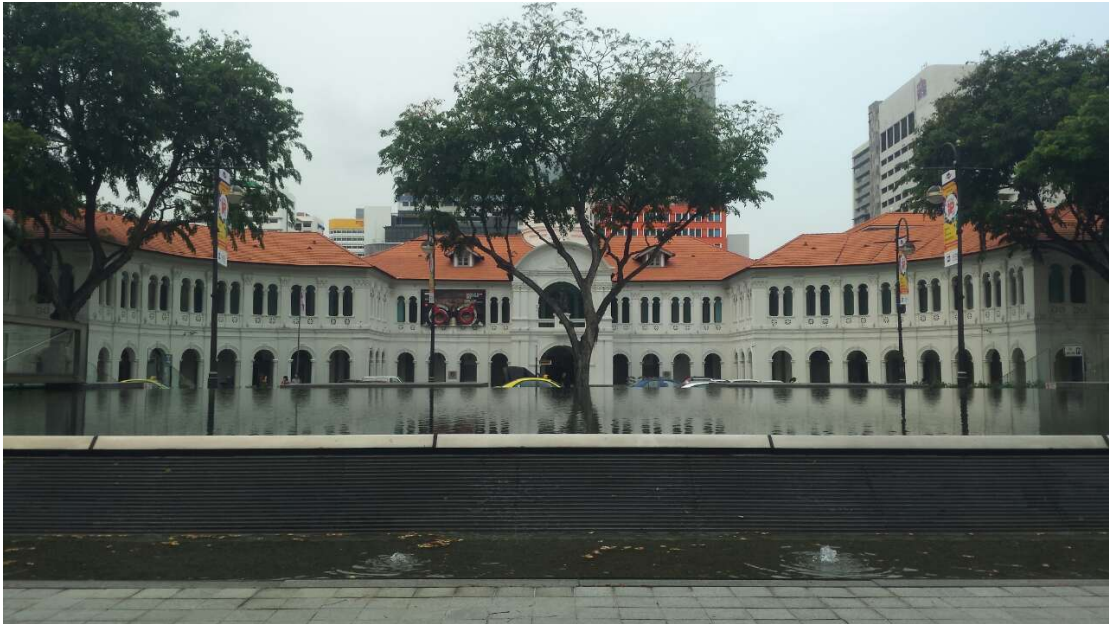
Figure 21 A building in Singapore
